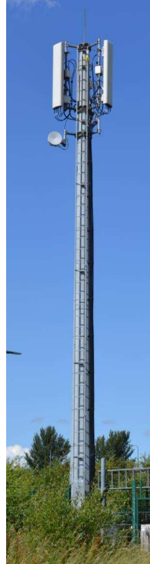
Dual band cross polarisation (polarisation diversity)
