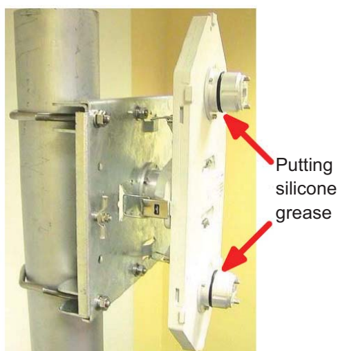
Figure 550. Putting silicone grease on O-ring before MPT-MC insertion (7-8 GHz)
