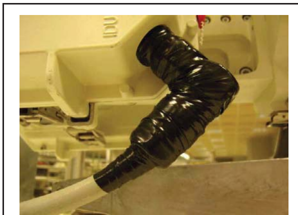
Surround the connector with the adhesive UV tape from up to down
