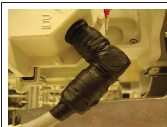
Surround the connector with the auto amalgamate tape from up to down
