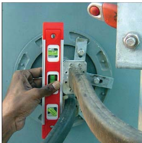
Figure 556. Checking Feedhead Flange with a Spirit level
