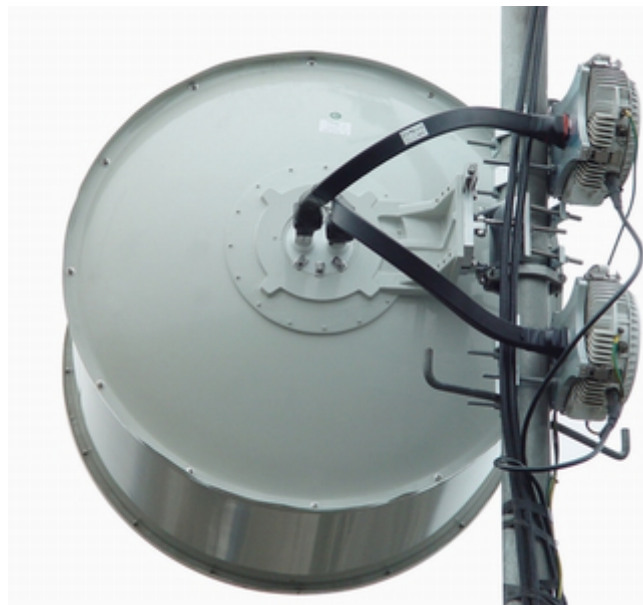
Figure 1-2 Separate mounting
