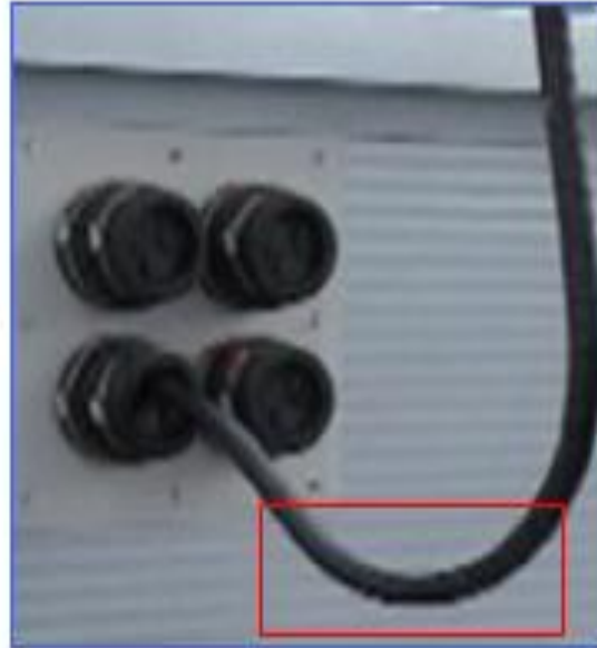
Make the waterproof curve
