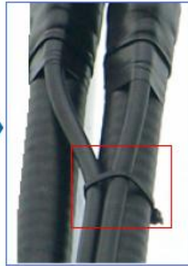
Bind the grounding cables
