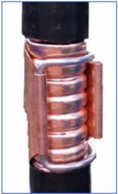
Install the metal jacket
