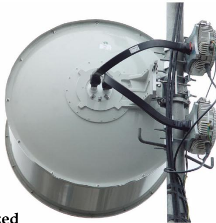
One ODU with One Antenna (Direct Mount)
