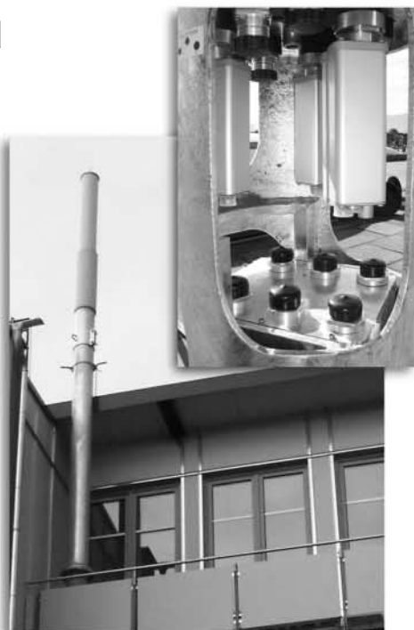
UMTS site of the operator T-Mobile in Germany with Kathrein's new Tri-sector pipe antenna and integrated RET system (new slimline RCUs) and TMAs.
